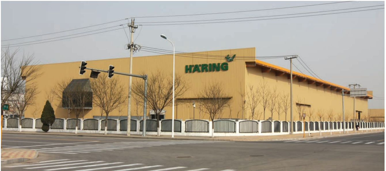
Häring factory, Tianjin (China)
